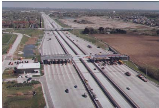
Figure 2-2: Sample Barrier and Ramp Plazas
